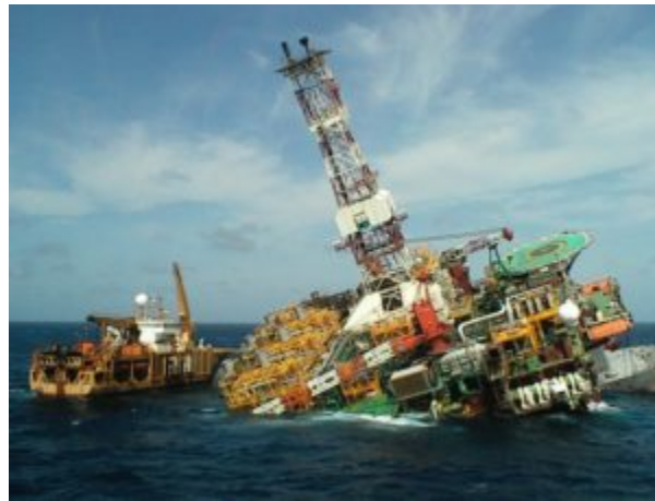
Figure 2.4.: The Petrobras P-36 oil platform sinking.
