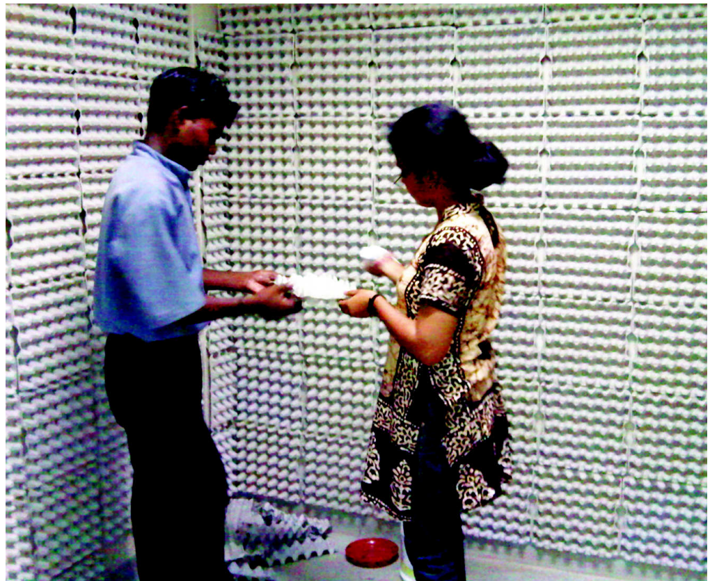
Figure 5.9: Egg tray covered walls in Gurgaon Ki Awaaz CRS, Gurgaon Photo courtesy: N.Ramakrishnan/Ideosync
